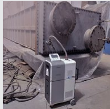
Heat exchanger detection
